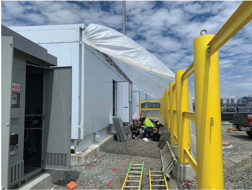
Testing N crane power switch gear
