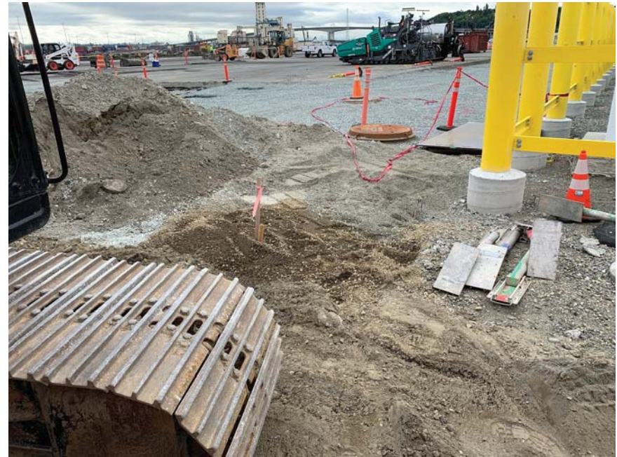
N Marine Building – Sanitary Sewer Backfill
